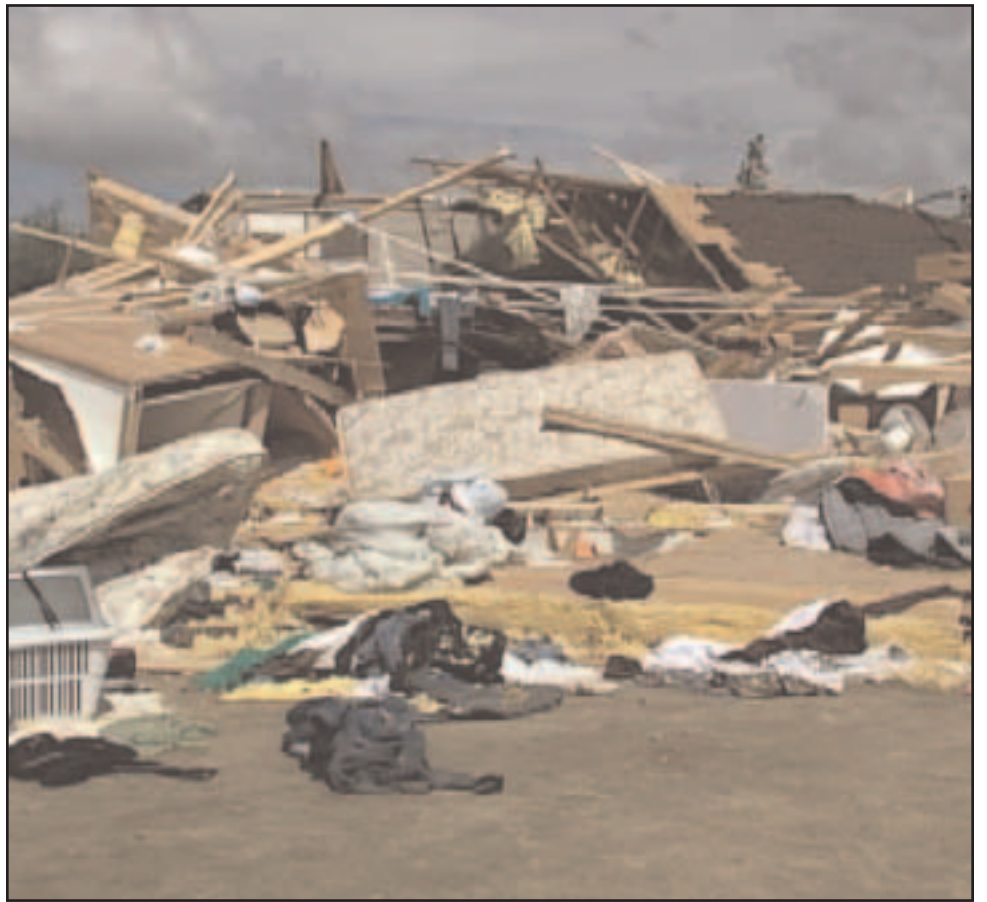
More than a dozen homes were destroyed or damaged and 80 people are homeless.
